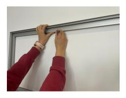
1. Place the frame against the wall. Position the bracket(s) evenly to ensure a well-distributed mounting system to support the weight and position of the frame securely onto the wall.
