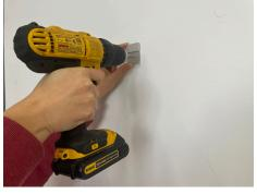
2. Attach the bracket(s) onto the wall by fastening the screws adapted to your wall. For a gypsum wall, we suggest to use plastic anchors before fastening the screws to secure the frame to the wall.
