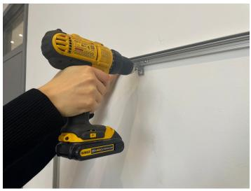
2. Attach the frame onto the wall by fastening the screws adapted to your wall into the bracket(s). For a gypsum wall, we suggest to use plastic anchors before fastening the screws to secure the frame to the wall.
