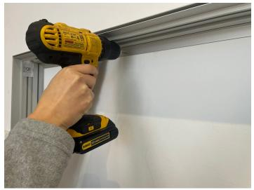
**2.** Attach the frame onto the wall by fastening the screws adapted to your wall into the frame's perimeter. For a gypsum wall, we suggest to use plastic anchor prior.
