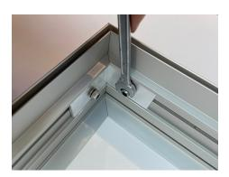
**3.** Assemble all the frame, then securely screw each junction using the Ratchet wrench.
